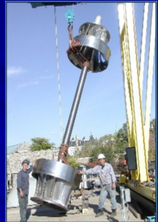
Replacement Francis Runners Ottawa Hydro
