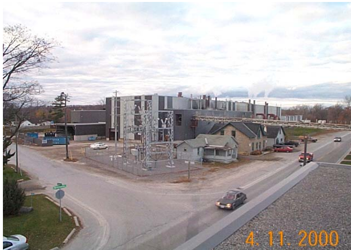
SONOCO Trenton 6 MWe CHP Plant
