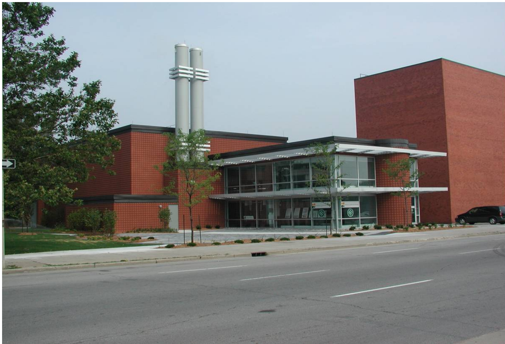
Hamilton District Energy ( 3 MWe) (FVB Energy)
