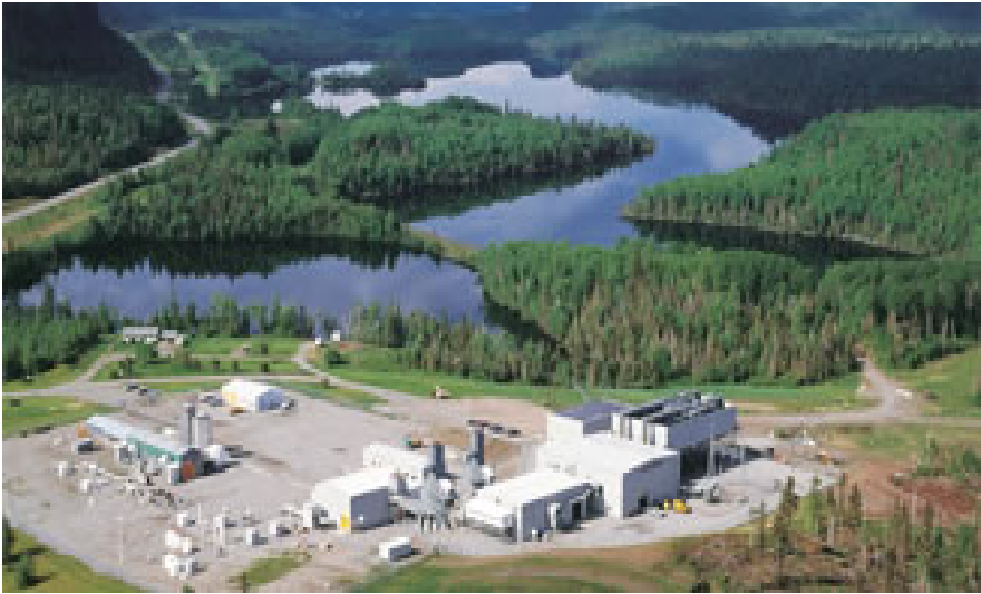
TCPL Nipigon 40 MWe Enhanced Combined Cycle
