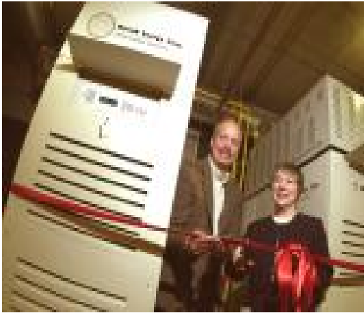
Capstone Microturbines SAIT, Calgary
