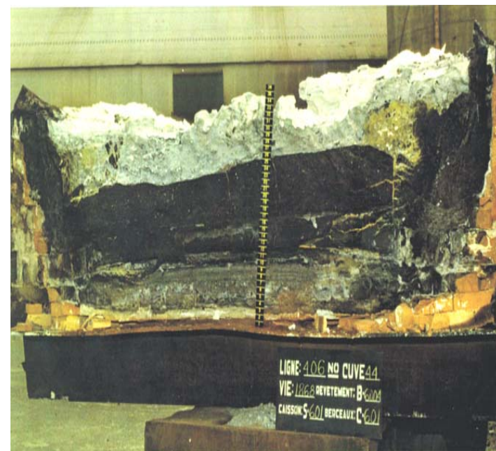
Cross section of potshell showing layers of refractory brick (red) and SPL (black)
