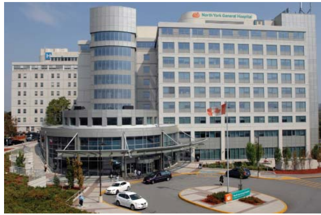
North York General Hospital.
